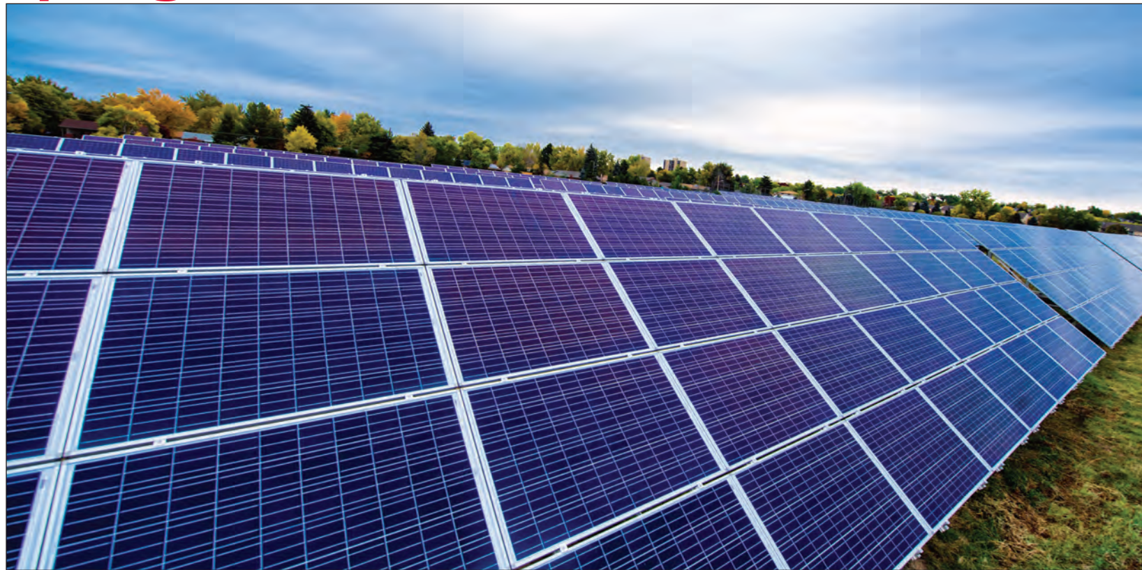
This year, Xcel Energy more than doubled the amount of energy under contract in its Solar*Rewards® Community® program, or solar gardens.
