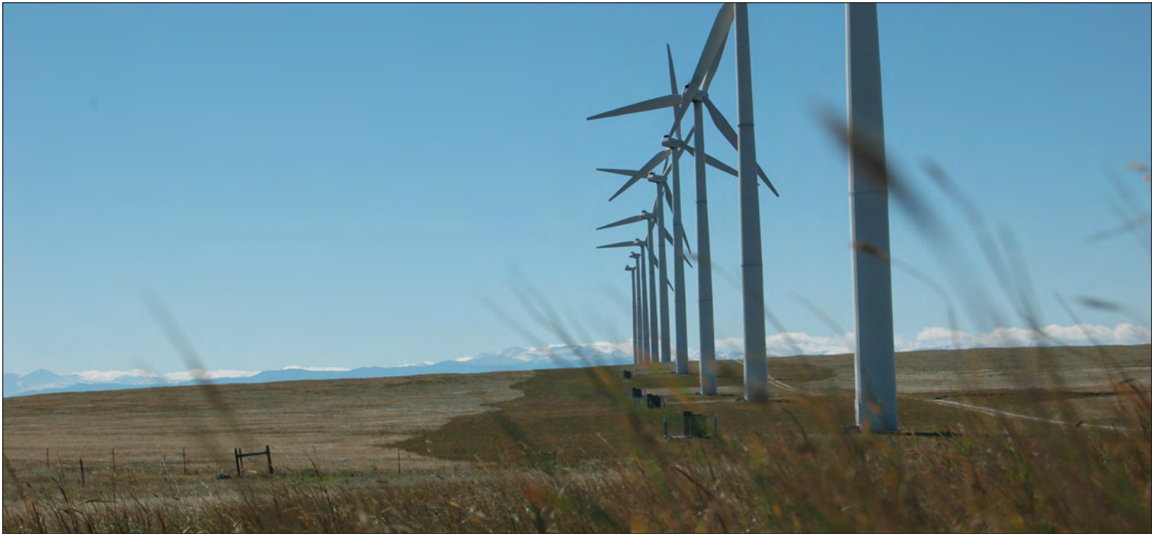
Today, 22 percent of the electricity on Xcel Energy's system in Colorado comes from renewable resources. (Xcel Energy)
